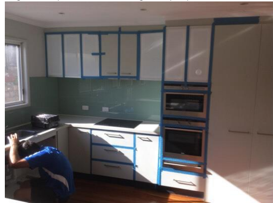
Taping and securing of cupboards to prevent dust
