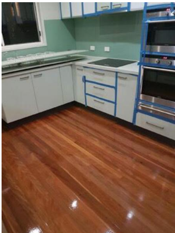
First coat finished
