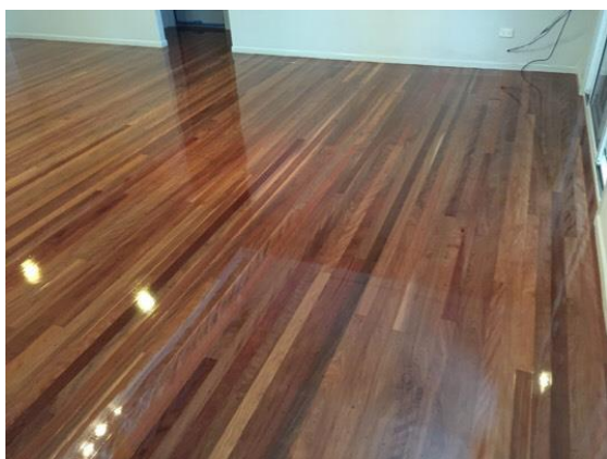
High gloss timber floor after repair
