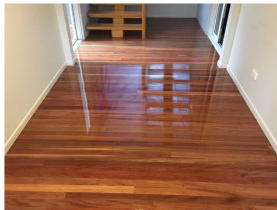
High gloss timber floor after repair
