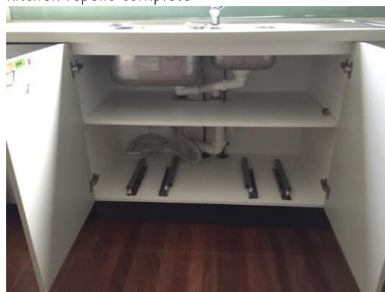
Repairs completed under sink
