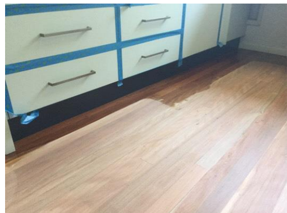
First coat being applied
