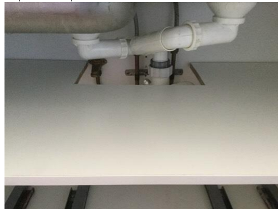
Close-up of completed repairs for insurer
